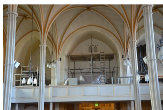
Painting the arches during restoration
